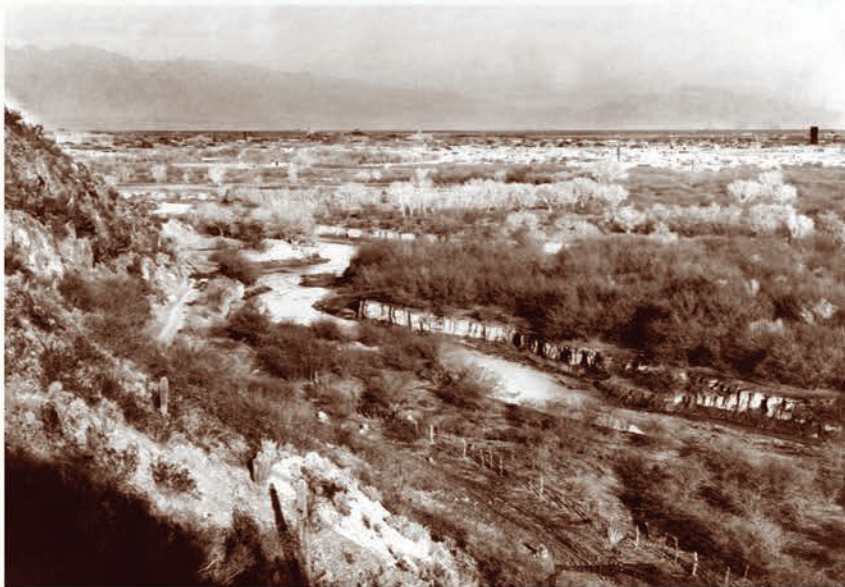
Left: This photograph of the West Branch (the channel in the foreground) and the Santa Cruz proper (channel not visible in the photo), taken from A Mountain in 1904, near the current intersection of Mission Road and 22nd Street, shows the headcut resulting from Sam Hughes' ditch. The remnant of an old dam can be seen left of center, just upstream from what was then the confluence of the mainstem and West Branch. (Walter Hadsell, 24868, courtesy of the Arizona Historical Society.) Right: By 2000, the West Branch was engineered to join the Santa Cruz channel further upstream, and the river channel was locked in place with soil cement. (D. P. Oldershaw, Stake 1026.)
