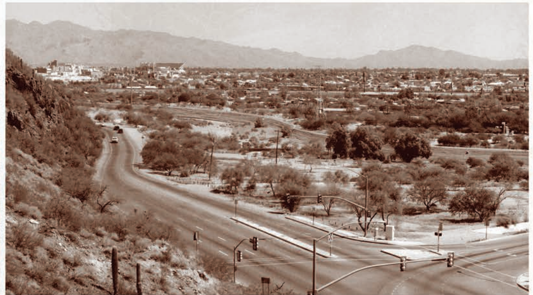
Left: This photograph of the West Branch (the channel in the foreground) and the Santa Cruz proper (channel not visible in the photo), taken from A Mountain in 1904, near the current intersection of Mission Road and 22nd Street, shows the headcut resulting from Sam Hughes' ditch. The remnant of an old dam can be seen left of center, just upstream from what was then the confluence of the mainstem and West Branch. (Walter Hadsell, 24868, courtesy of the Arizona Historical Society.) Right: By 2000, the West Branch was engineered to join the Santa Cruz channel further upstream, and the river channel was locked in place with soil cement. (D. P. Oldershaw, Stake 1026.)
